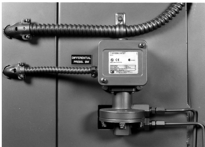
FIGURE 19 - DIFFERENTIAL PRESSURE SWITCH
